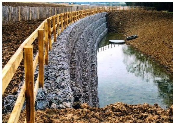
Figure 6 Gabion retaining wall [11]
