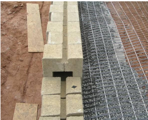
Figure 3 Segmental block retaining wall [11]
