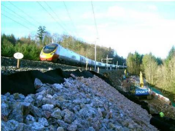
Figure 24 Bessy Gill railway embankment stabilisation [8]
