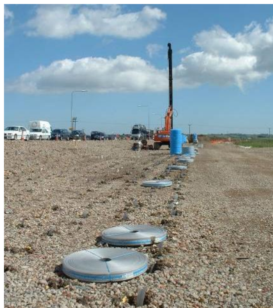
Figure 32 PVD geocomposites provide effective ground improvement solutions [8] & [4]
