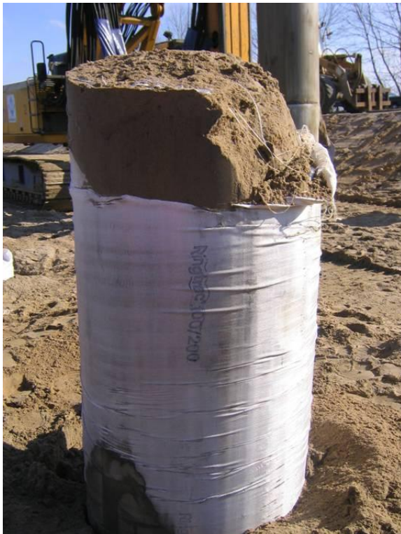
Figure 10 Geotextile encased column [9]
