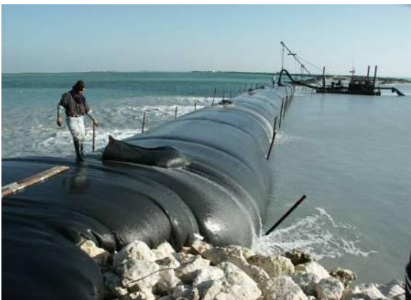
Figure 13 Geotubes used for coastal erosion and sludge drainage applications [18]
