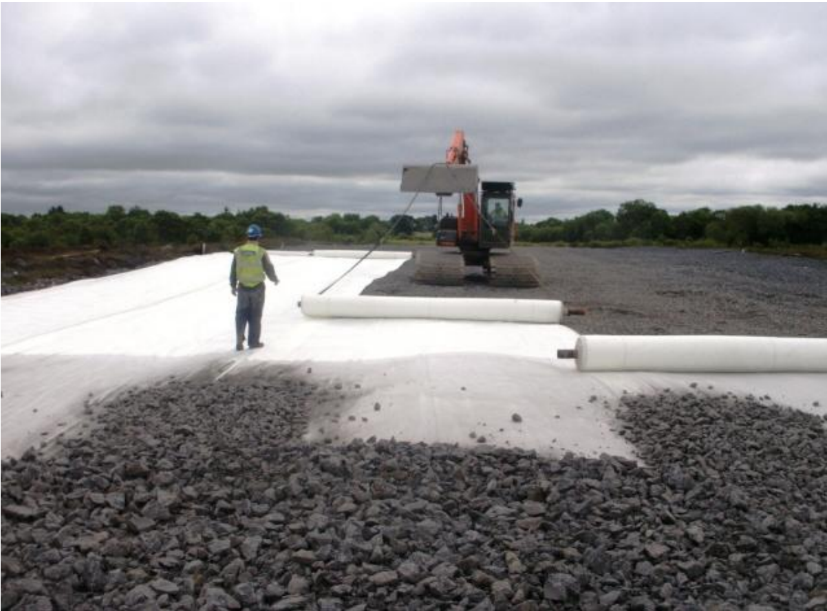
Figure 34 Basal reinforcement and a 6C stone drainage layer being installed to enable future construction of road embankments [9]
