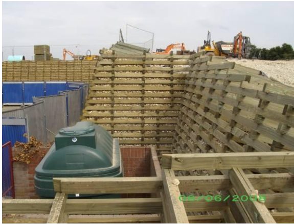
Figure 4 Timber crib retaining wall [15]
