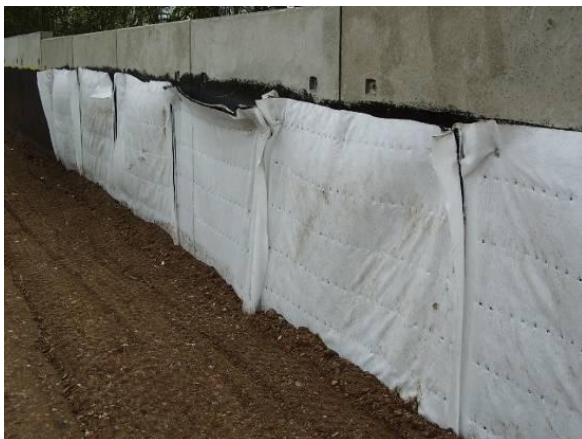
Figure 38 Drainage Geocomposite; M25 Widening [12]
