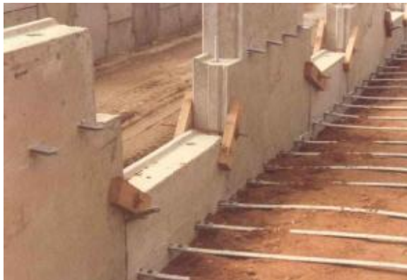
Figure 8 Steel strip reinforced wall system [17]
