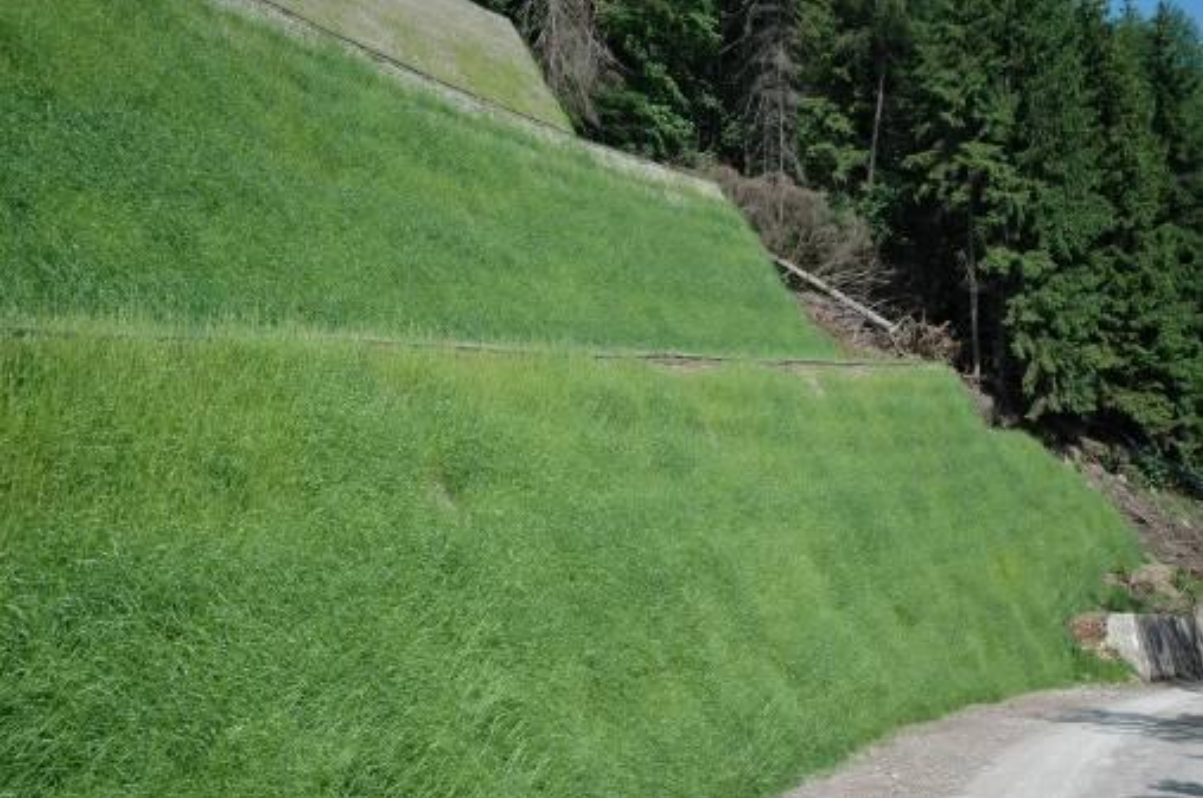
Figure 28 Gabion and Crib gravity walls An example of a vegetated reinforced soil slope [9]
