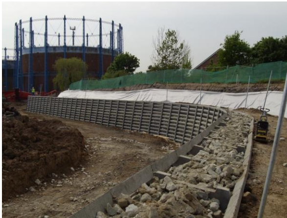
Figure 30 Concrete Crib gravity retaining wall [15]
