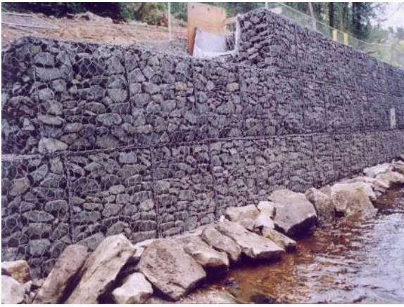
Figure 1 Gabion retaining wall [11]
