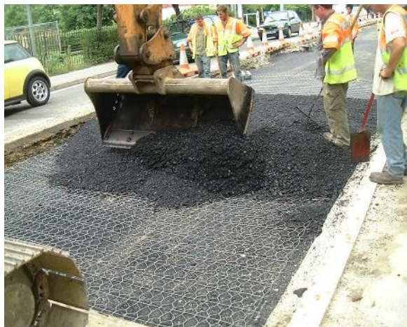
Figure 37 Steel mesh reinforcement being used on Abingdon Road, Oxford [11]
