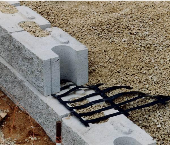
Figure 16 Block and geogrids [11]
