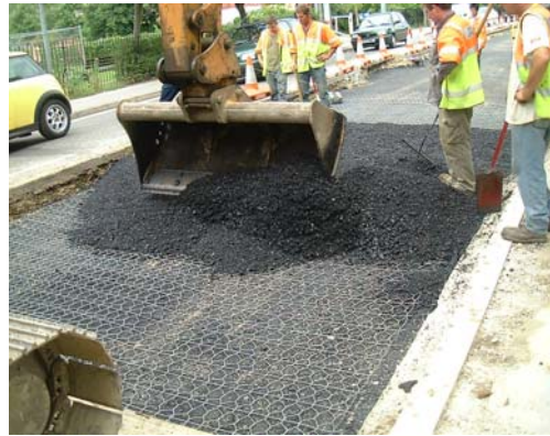
Figure 1: Reconstruction in progress (Photograph courtesy of Maccaferri Ltd)
