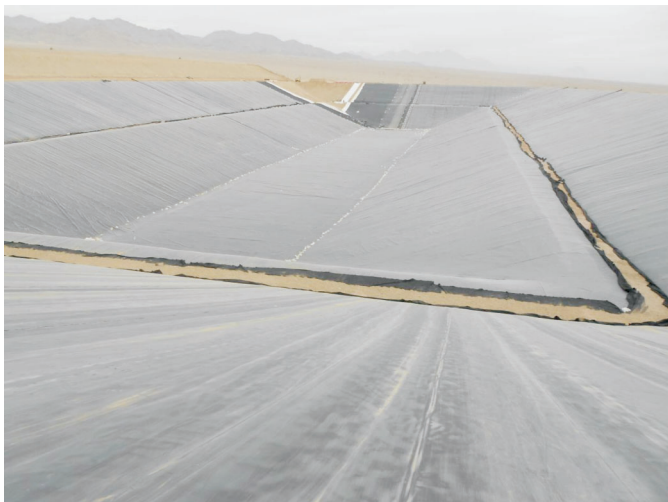
Geosynthetic Liner Deployment Nearing Completion
