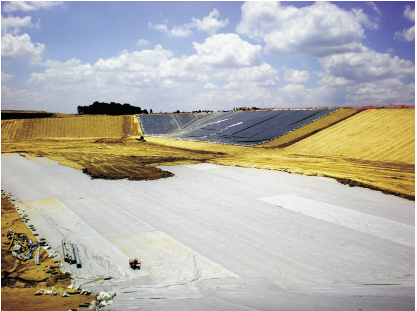
Construction of a hazardous waste cell
