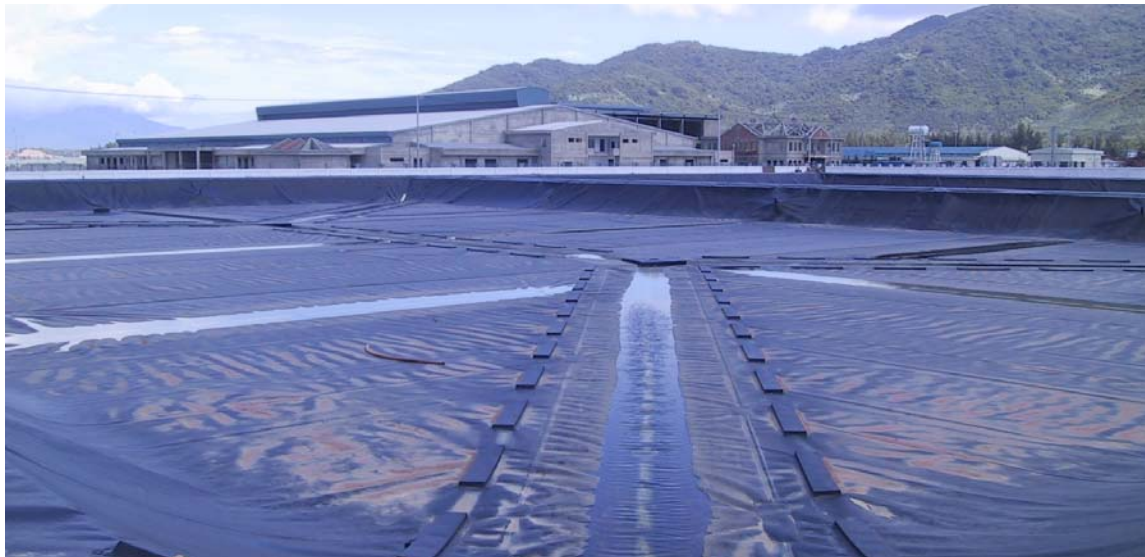
Fig 6. An Anaerobic wastewater processing facility with floating cover and gas collection
