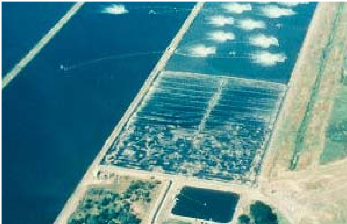
Fig 10. A combined anaerobic and aerobic system as part of a much larger system
