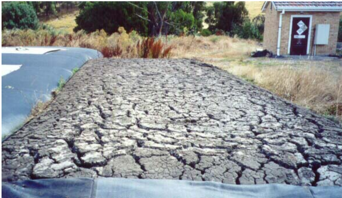
Fig 11. Dried sludge from a geotextile sludge dewatering bag
