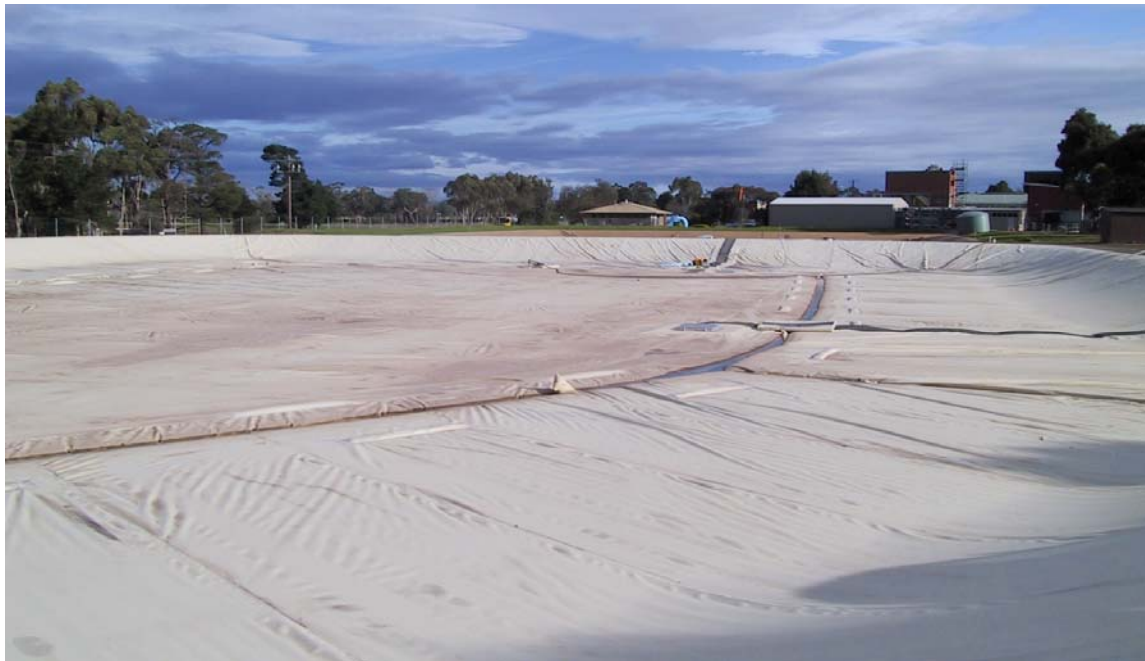
Fig 3. A floating membrane cover to a water storage facility
