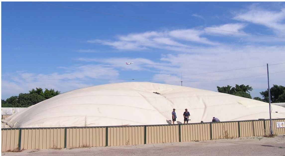
Fig. 4 Geomembrane bladder for water and gas storage
