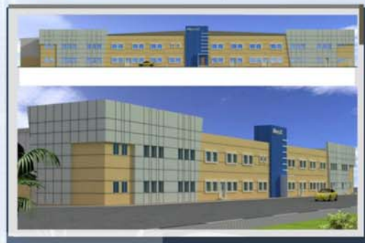
Mattex Jubail–Nonwoven (under construction)
