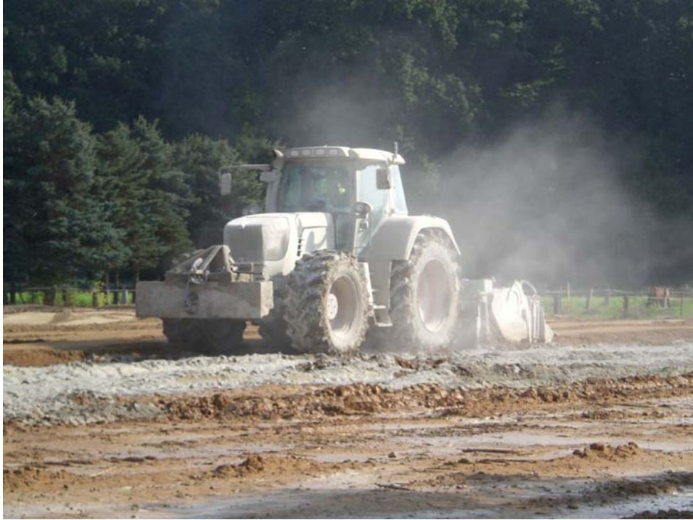
Fig. 7: Example of base soil improvement by milling of binder (lime/cement) into the soil
