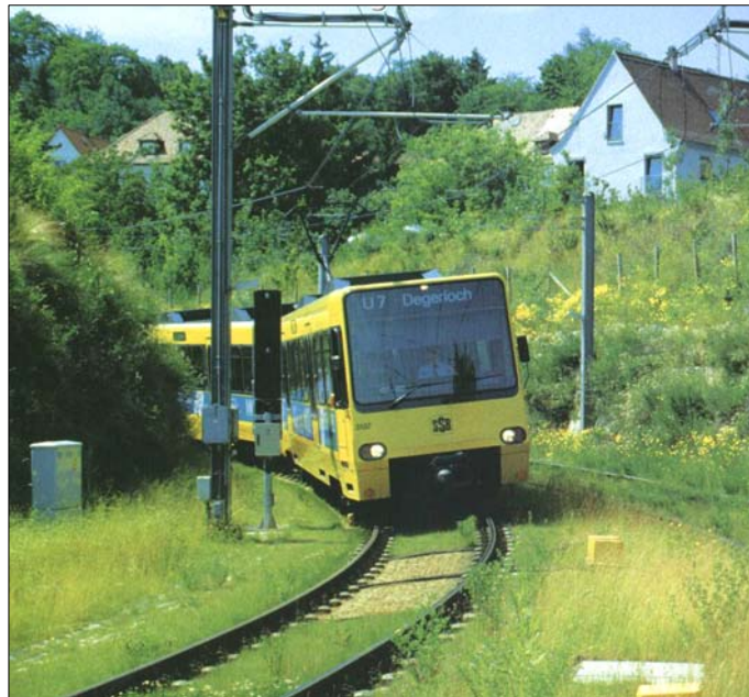
Fig. 1: City railway Stuttgart, Germany. Example of a greened up geogrid reinforced supporting structure (1990)
