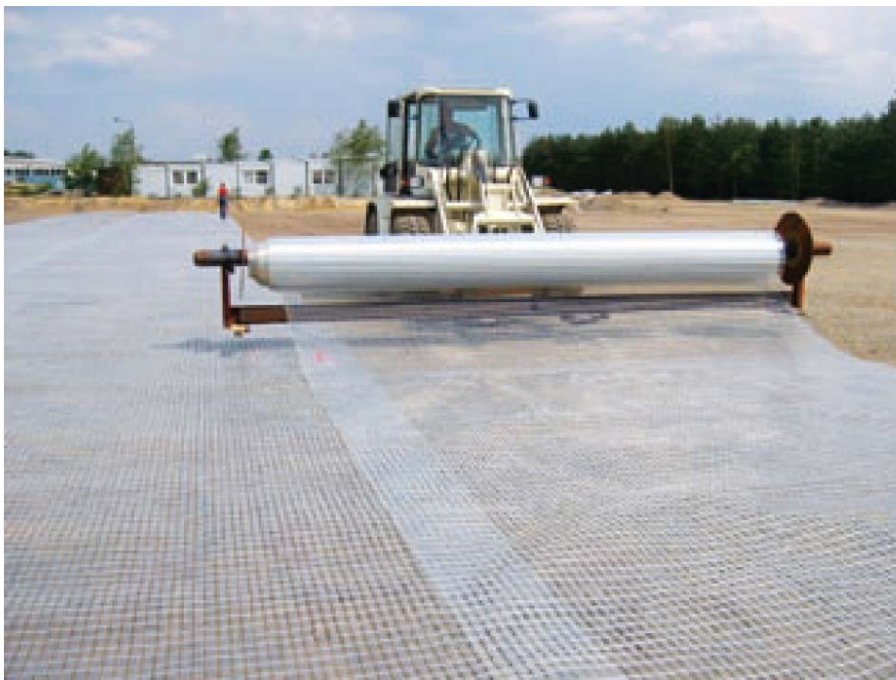
Fig. 8: Example for base soil reinforcement with a biaxial polypropylene geogrid
