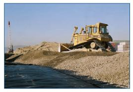
*Mirafi® HP570 provides subgrade stabilization and base reinforcement.*
