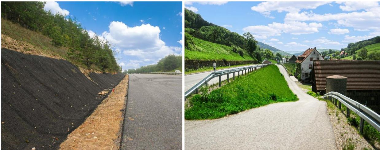
Figure 7: a. Motorway embankment in construction stage b. Road embankment with erosion control
