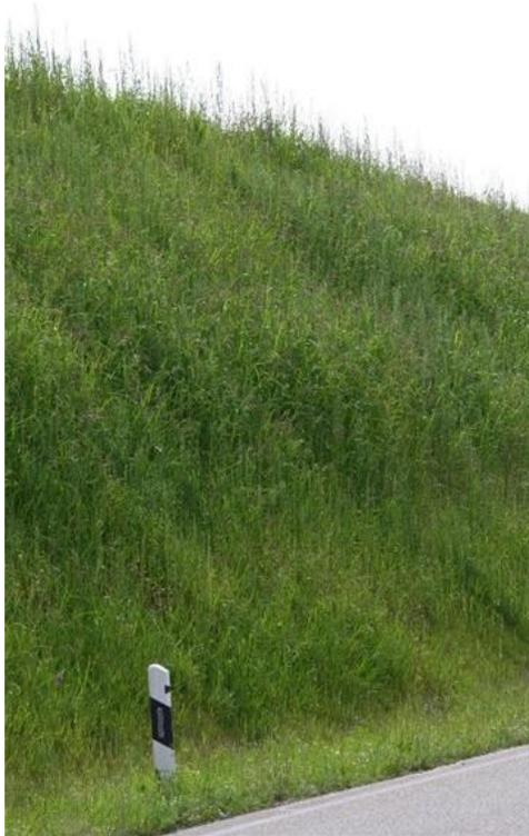
Figure 1: Vegetated, erosion control on road embankment
